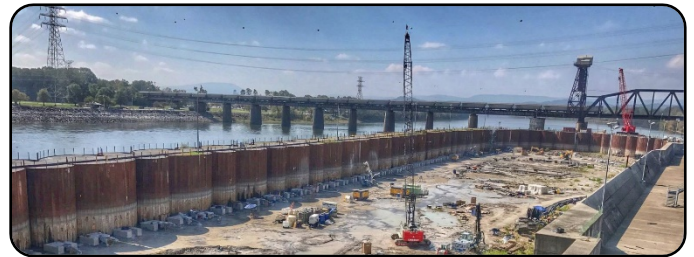
USACE Chickamauga Lock Excavation
